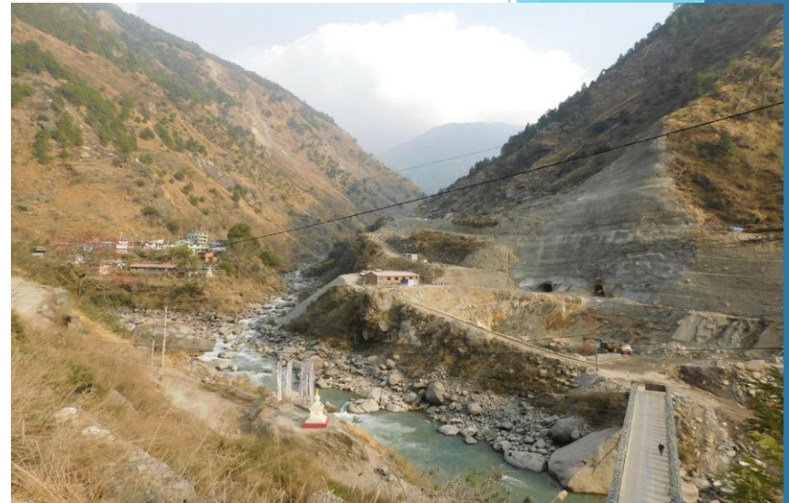
Hydropower project at Syabrubesi Bazaar, Rasuwa
